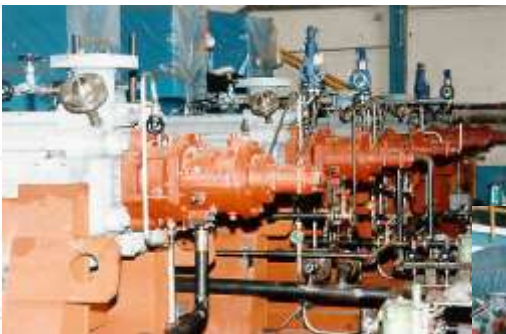
Boiler Feed Water Pumps with Oil-system 0.9 MW for Combined-cycle Power Plant Tambak Lorok
