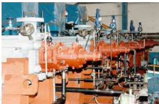
Boiler Feed Water Pumps with Oil-system 0.9 MW for Combined-cycle Power Plant Tambak Lorok
